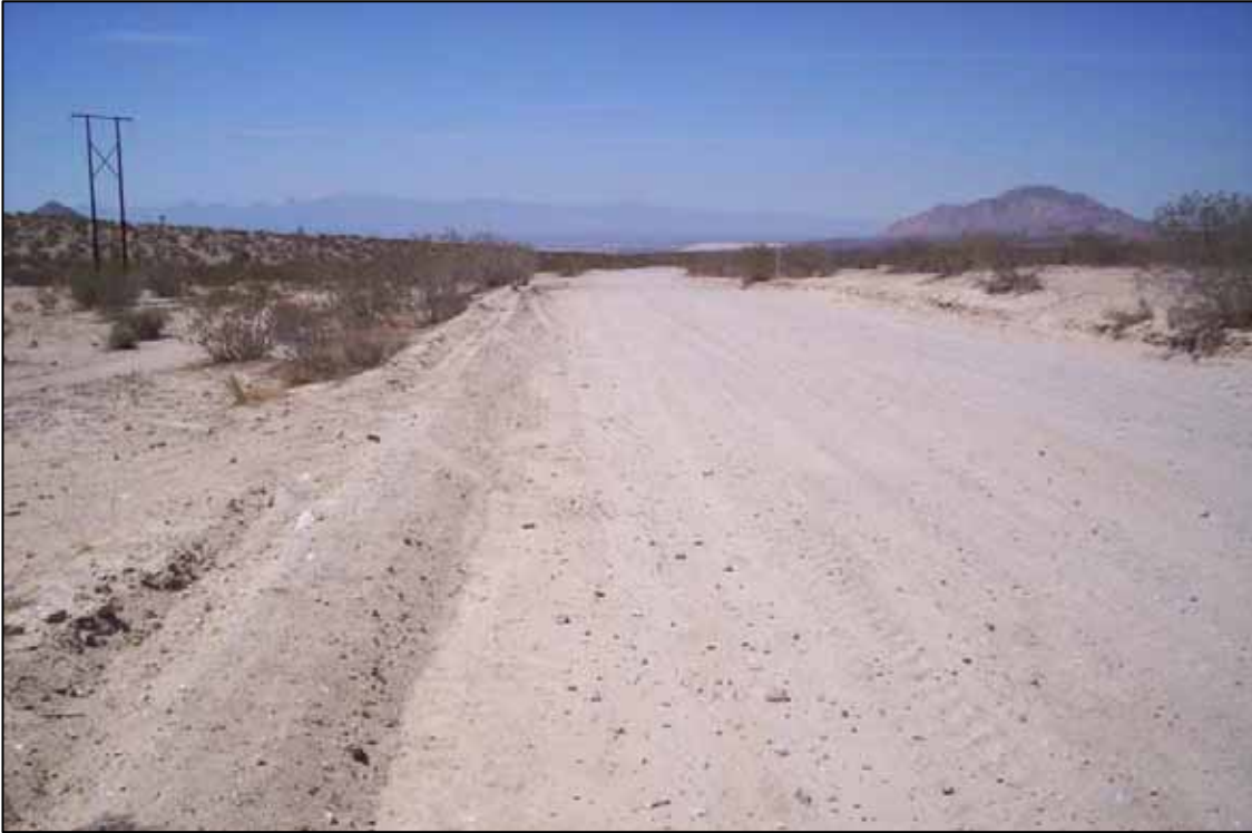
Photo 7. Photo taken along Segment 3 looking southwest towards the I-15. The width of the road is approximately 30-feet, with a small amount of shoulder vegetation within the berms of the road.
