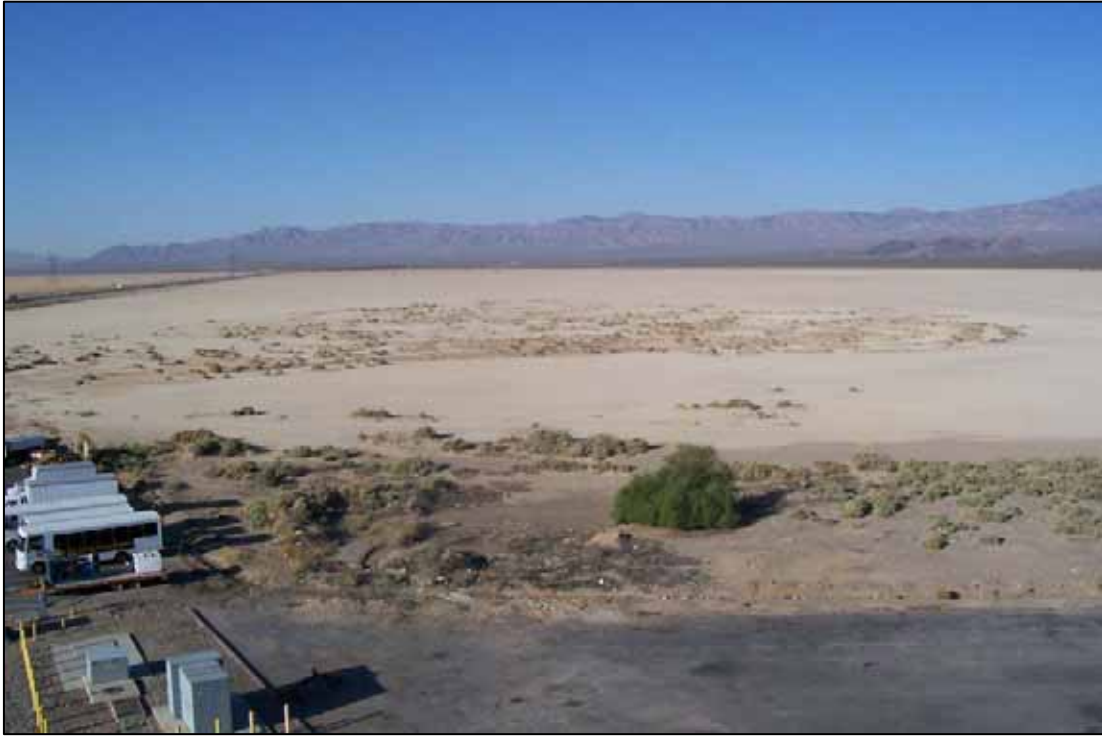
Photo 1. Photo taken from CA-NV state line at Whiskey Pete's parking lot looking south at the dry Ivanpah Lake bed. The cable route (Segment 1) lies parallel to the I-15 on the left side of the photo then crosses the lakebed along the utility corridor.
