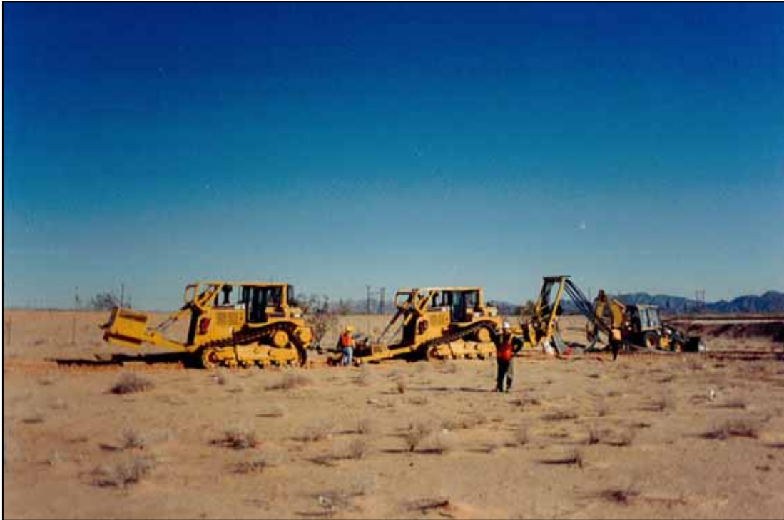
Photo 9. Photo depicts representative construction equipment for installation of multiple conduit lines during Level 3 fiber optic line installation; however, AT&T proposes one conduit line. Bulldozer at far left, trench/plow rig in center, and backhoe far right.
