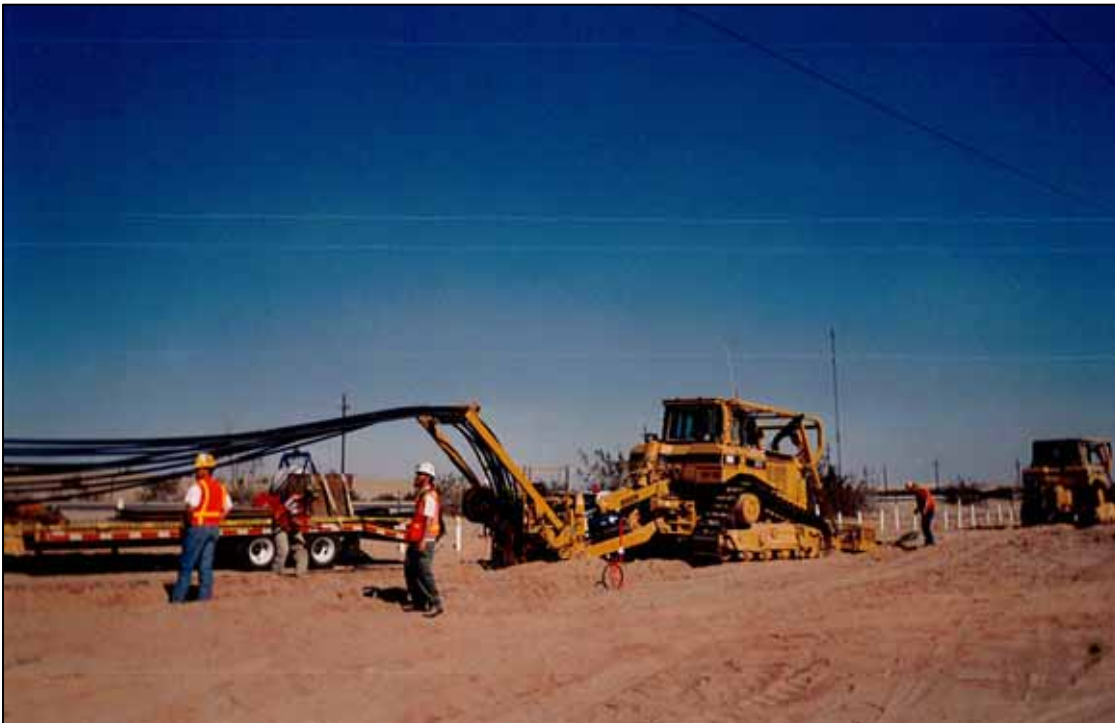
Photo 9. Photo depicts representative construction equipment for installation of multiple conduit lines during Level 3 fiber optic line installation; however, AT&T proposes one conduit line. Bulldozer at far left, trench/plow rig in center, and backhoe far right.
